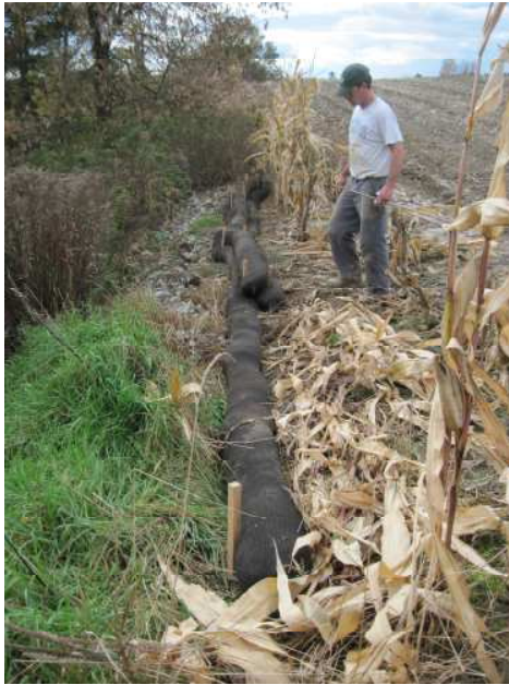
Compost filter socks will prevent field runoff from reaching Rock River
