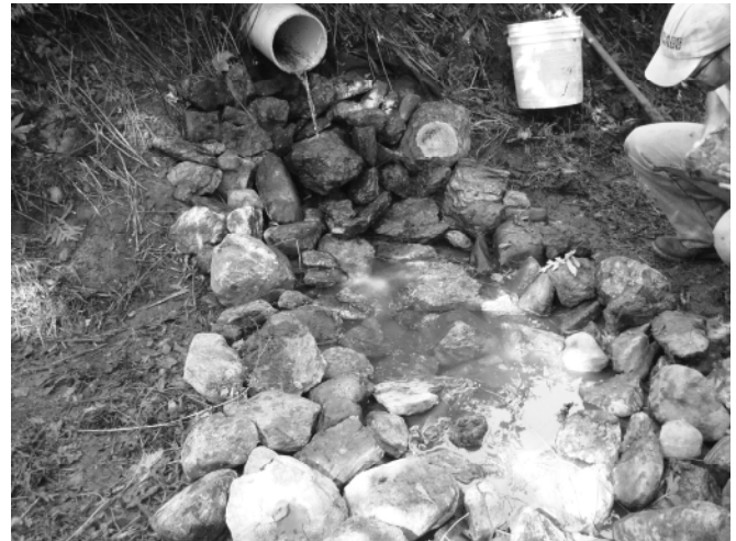
Soil erosion is reduced by lining a culvert outlet with fabric and stones
